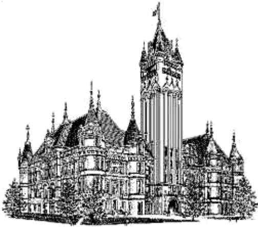
SPOKANE COUNTY COURT HOUSE
